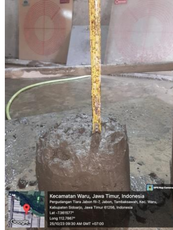
Gambar 3. Hasil Uji Slump Beton
